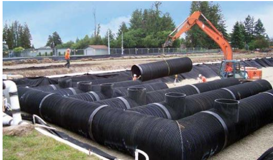
Figure 1. Example of a Subsurface Detention Gallery
