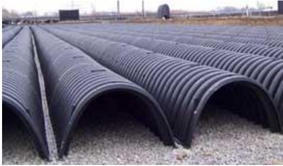
Figure 1. Example of a Subsurface Infiltration Gallery
