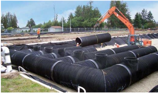
Figure 1. Example of a Subsurface Detention Gallery
