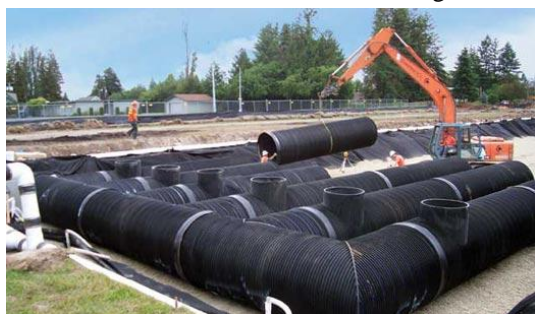
Figure 1. Example of a Subsurface Detention Gallery
