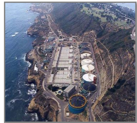
Savings at the Point Loma Plant. Avoided costs at the Point Loma Plant played an important role in establishing reuse targets. The land available at Point Loma Site is constrained, and any upgrades incur high costs.
