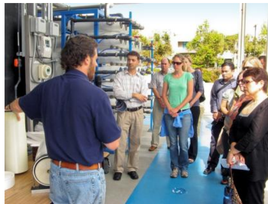
Public Utilities Department staff tour the AWP Facility.
