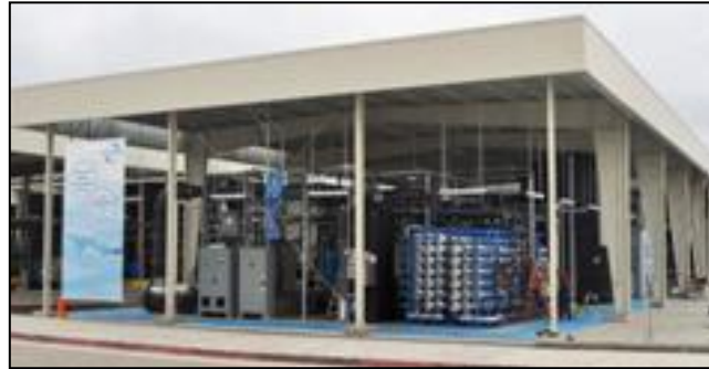
Figure 2-1. Water Purification Demonstration Project
