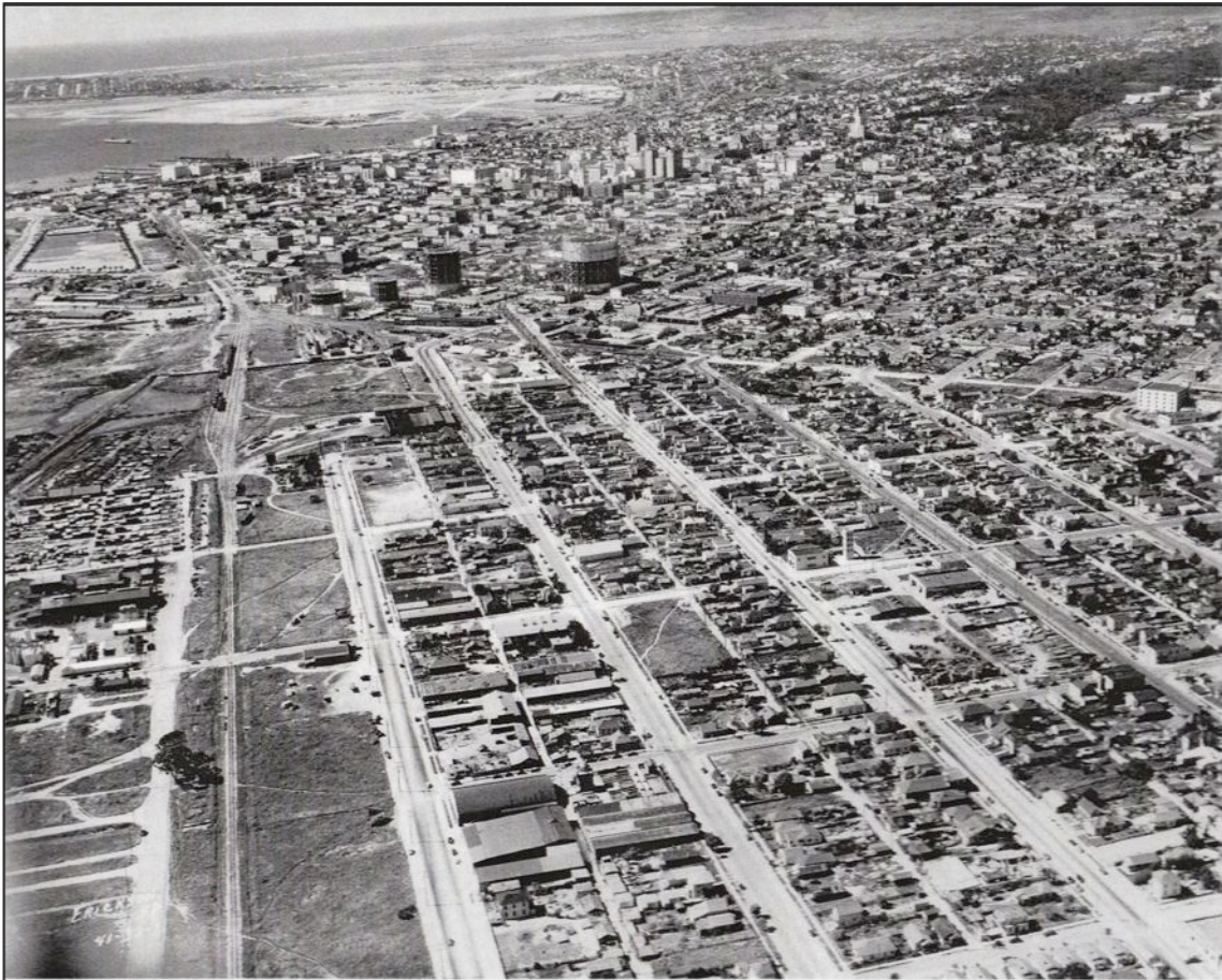
Plate 12. Close-up aerial photograph of the plan area during World War II, facing north. The railroad tracks are on the left side of the frame (left of Main Street). The dirt track to the left of the railroad tracks is Harbor Drive. Note the denseness of development at that time. Many of the buildings had outbuildings or second residences behind. Courtesy of SDHS.
