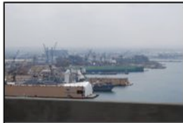
Plate 33. View of wharfs/docks from San Diego-Coronado Bay Bridge
