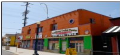
Plate 18. Bright paint on a commercial building, 2185-95 Logan Ave.
