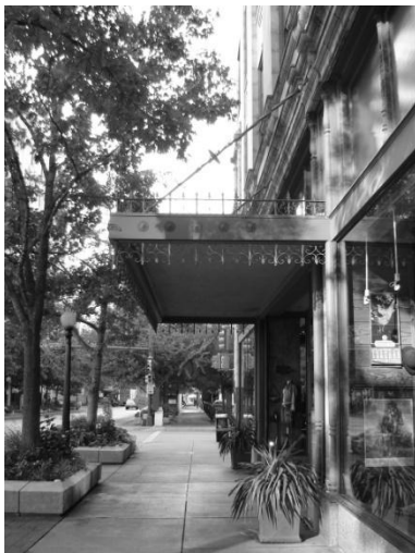
Entry Canopy and Planters
