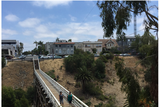
First Avenue Bridge
