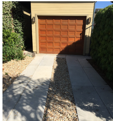
Residences can contribute to storm water filtration efforts by reducing the amount of impervious driveway areas.
