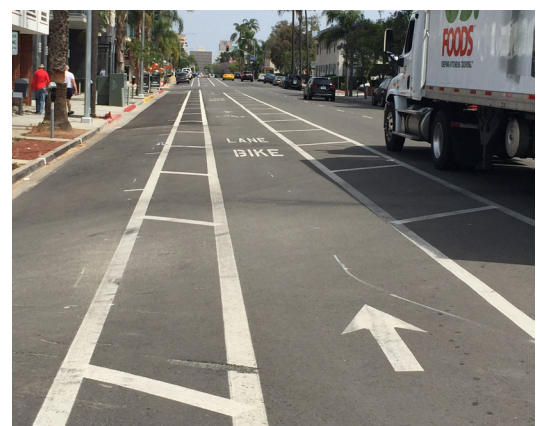
Buffered bike lanes along Fifth Avenue connect Downtown with Bankers Hill/Park West and Hillcrest.
