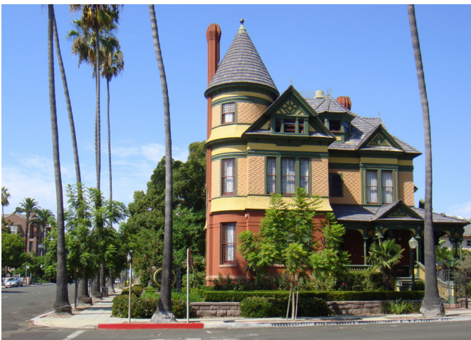
The Britt/Scripps House, built between 1887-1888, was renovated to become a boutique hotel, and is considered a model of adaptive reuse.
