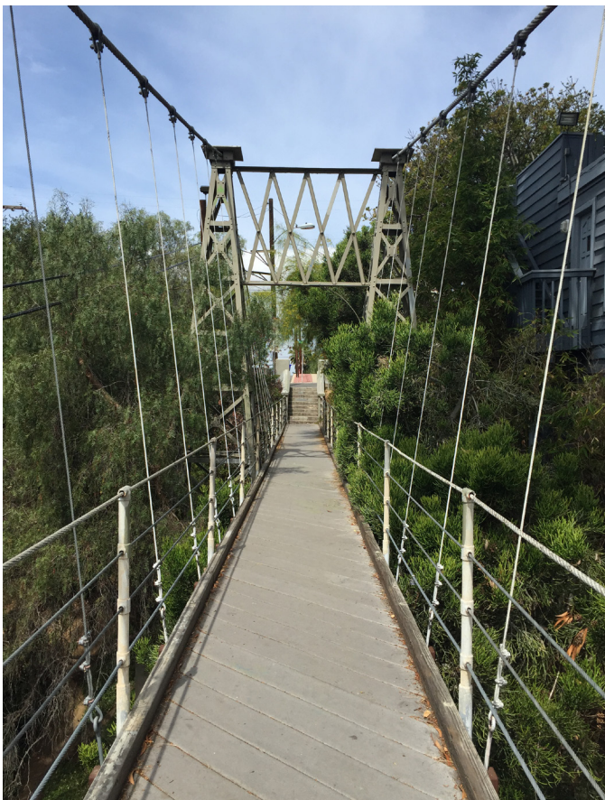
The Spruce Street Bridge, engineered by Edwin Capps, still provides access over Maple Canyon since its completion in 1912.
