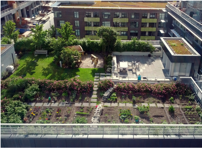
Rooftop gardens can serve a dual function of screening/obscuring rooftop mechanical equipment, and providing for on-site common space in urban areas.
