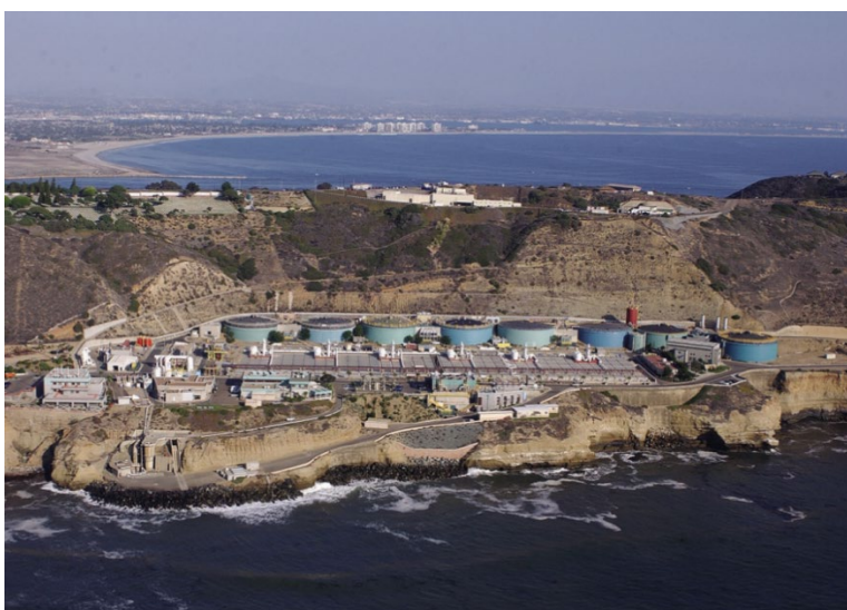
The Point Loma Wastewater Treatment Plant is the terminal treatment facility serving a Metro System population of approximately 2.2 million as of 2021.
